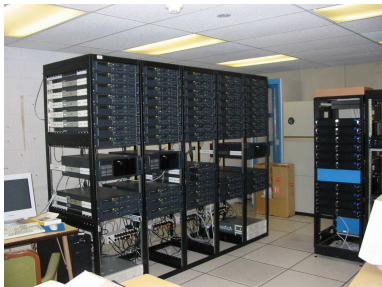
Keen Building, 3rd floor
